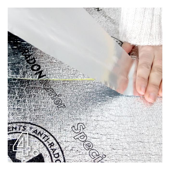
For sealing connections without an overlap (in the same row) use butyl/aluminium tape.
