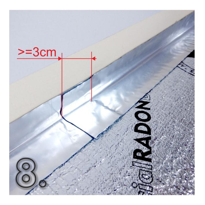
Make an overlap of minimum 3 cm on each connection of butyl tape if necessary.
