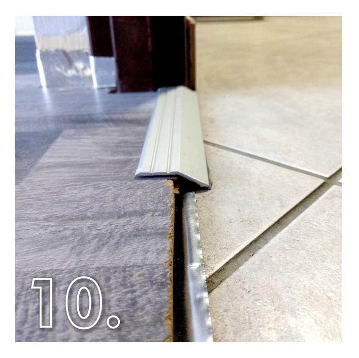
To ensure barrier layer integrity use only glued transition profiles. Avoid any perforation or damage of the Anti-Radon barrier layer.
