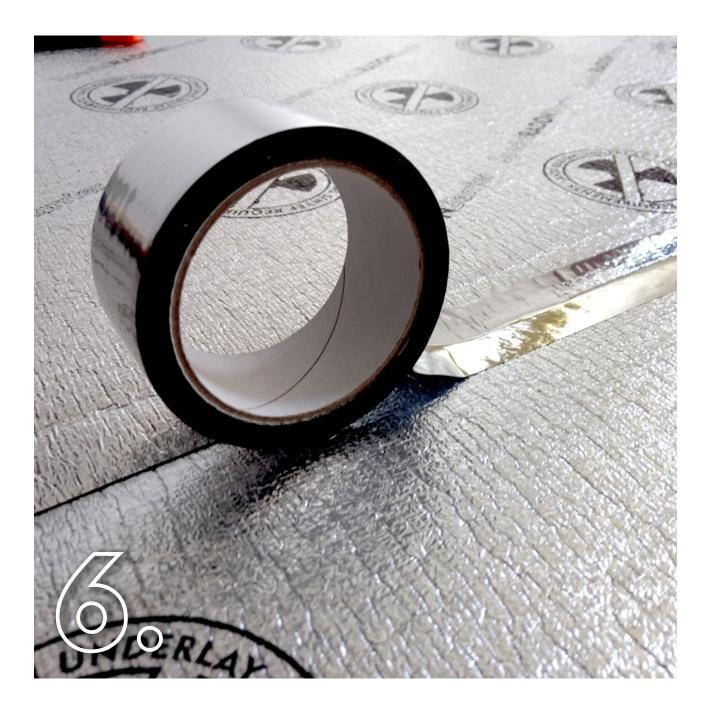
Seal the connections between paralell rows of underlay using aluminium sealing tape.
