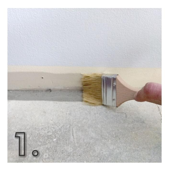
Ensure that all the floor/wall connections are clean, dust-free and pre-primed
