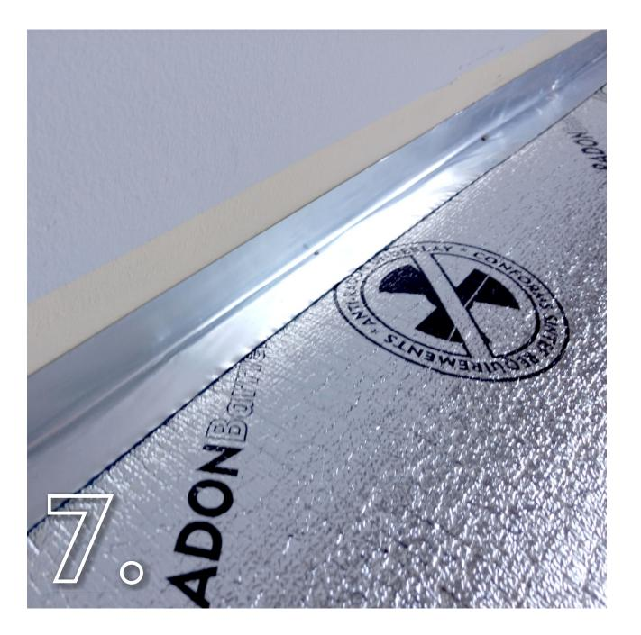
Seal all the edges of underlay running along walls with aluminium/butyl tape.
