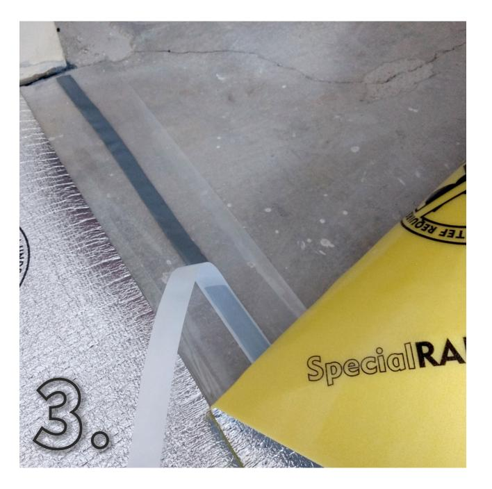
Seal paralell rows of underlay using overlap with butyl tape.
